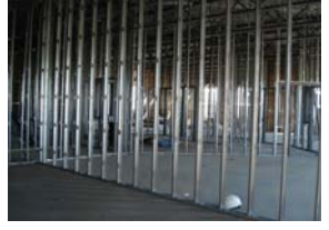
ADDITIONS & NEW CONST.
